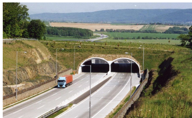
Figure 5: Overpass on the road R35 [13]
