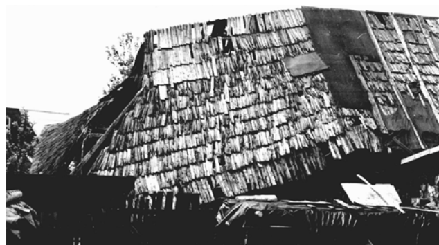
Figure 2: Wood shingle roof [2]
