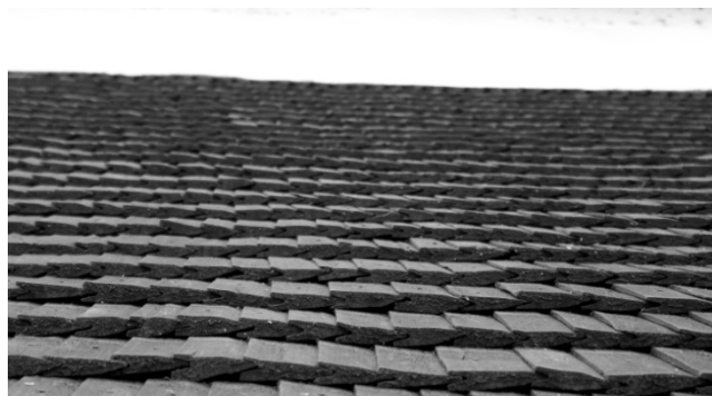
Figure 1 Traditional wood shingle roof, Church in Zehra
