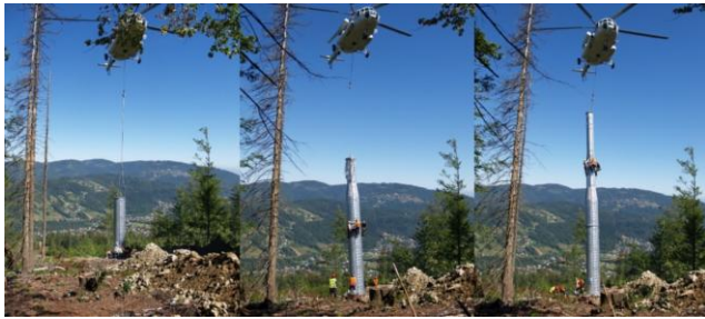
Figure 3: Stepwise assembly of the pipe-like shaft components of a tower (authors)
